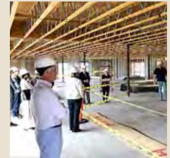
A media open house was held at the CF Campus during construction.
